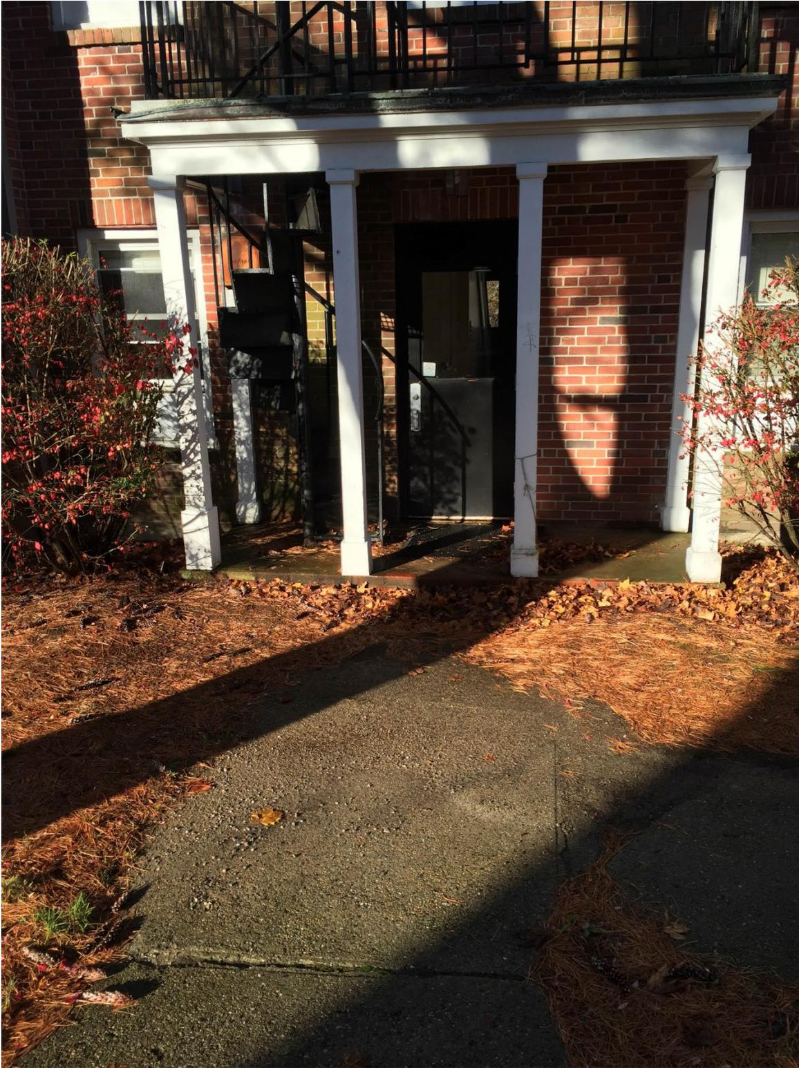
This feature contains a Concrete Ramp. There are Ramps/Walkways 5 feet wide and approximately 30 feet total length. | Total Area: 150 square feet.
